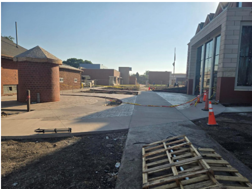
Stamped concrete complete.
