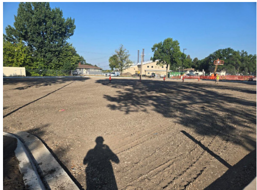
Parking lot ready for paving.
