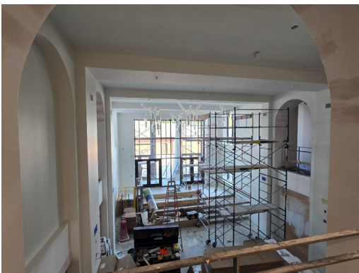
Lobby lighting installation underway.
