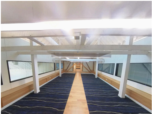
Final punch list work is underway on the fourth floor.
