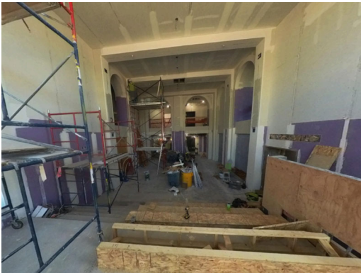
Lobby preparation is nearly complete and ready for paint.
