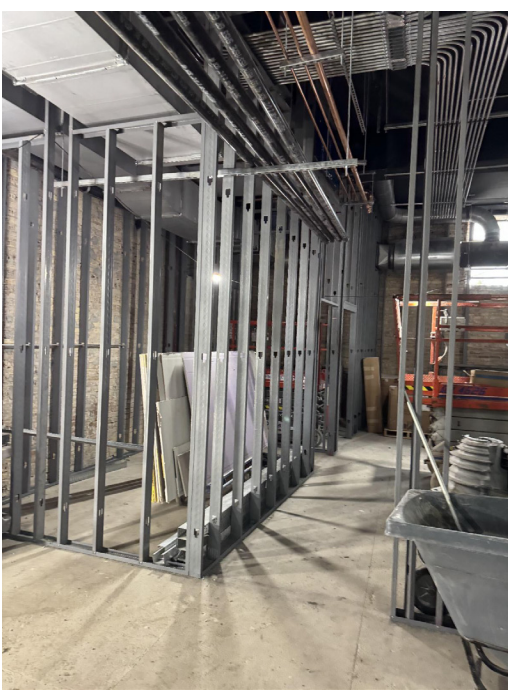
Theater Area: Wall framing nearing completion.
