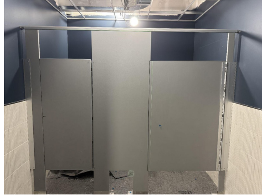
4th Floor: Bathroom partition installation in progress.
