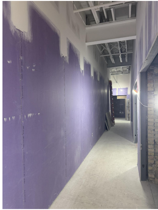
1st Floor – East Side: Sheetrock installation underway.
