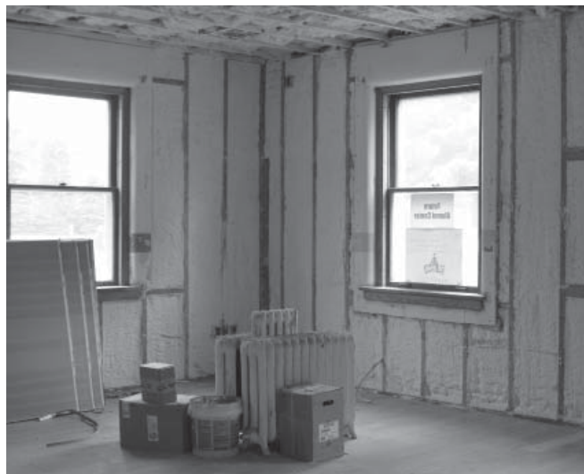
The brick walls were insulated prior to the installation of sheetrock.
