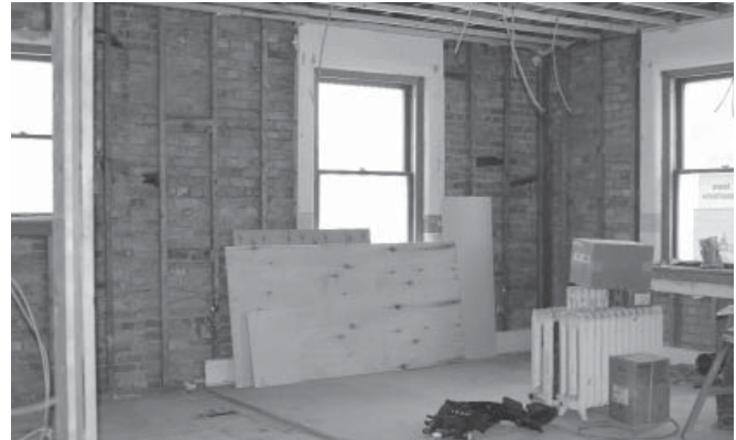
Interior demolition in June included removing the plaster walls and revealing the studs and the exterior brick walls.
